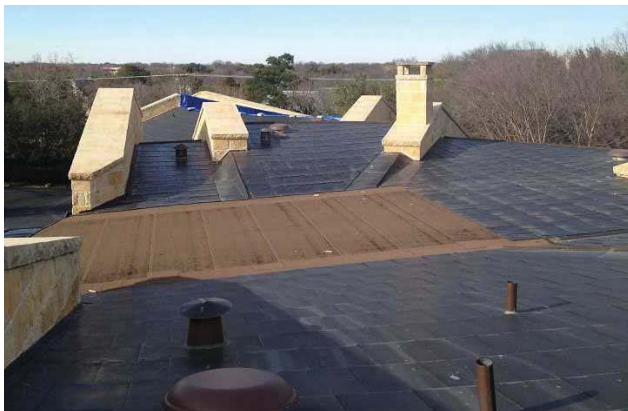
Most of the crew had never fabricated or installed tapered panels this long, so they were trained how to use New Tech's slitter and tapering equipment.
